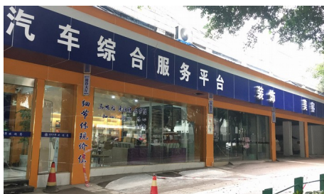
The Group’s service centre located at Longmatan Avenue in Luzhou City, which is a service centre only outlet
